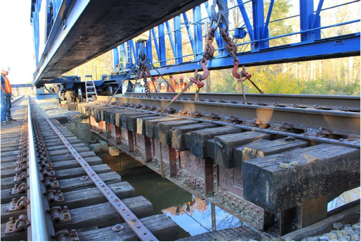
**Figure 8: Superstructure Removal**
