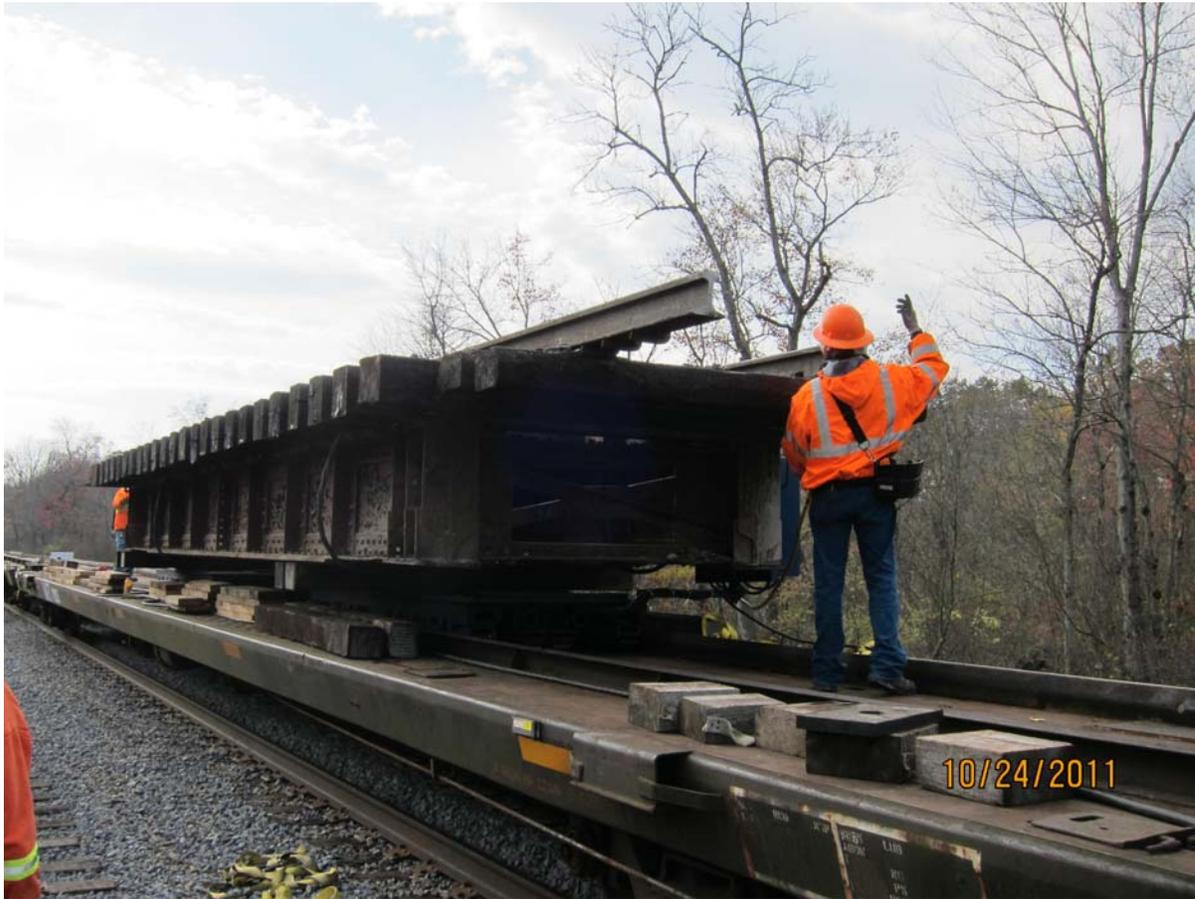
**Figure 10: Removal of Old Span**
