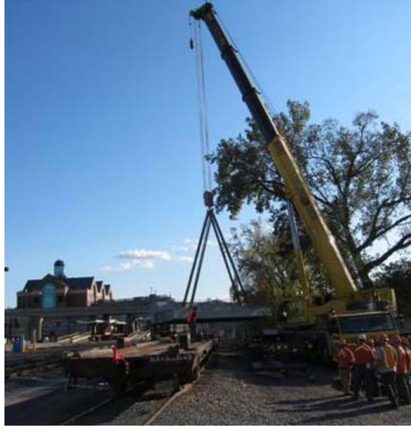
**Figure 5: 250 Ton Crane Loading Bridge Slabs on Flat Cars**
