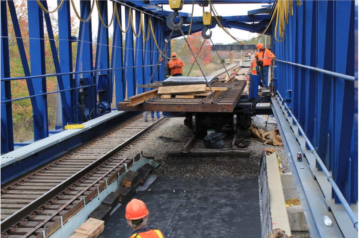
**Figure 12: Installation of Track Panel**
