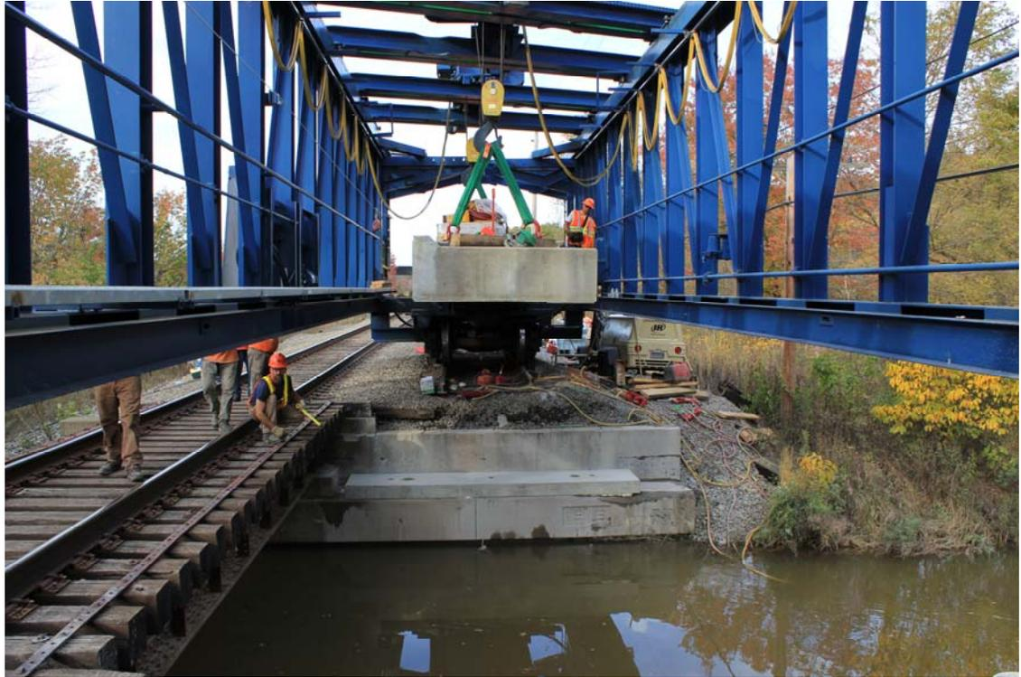
**Figure 9: Precast Bridge Slab Installation**
