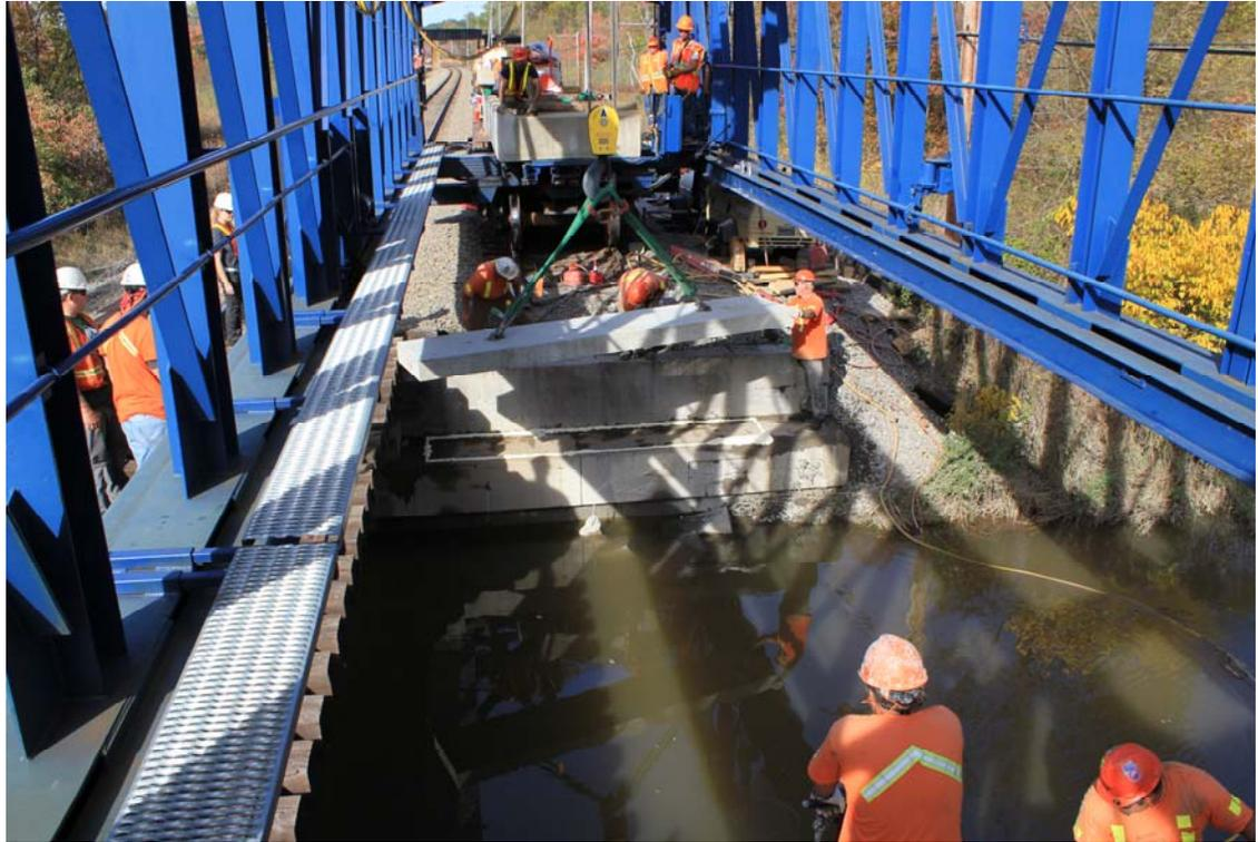
**Figure 11: Installation of Bridge Bearing Pad**
